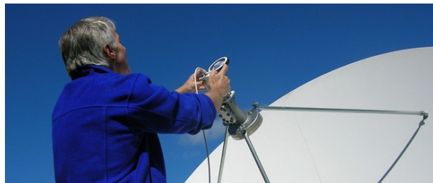
Martin Steinson adjusts the polarization angle of the LNB using a protractor.
