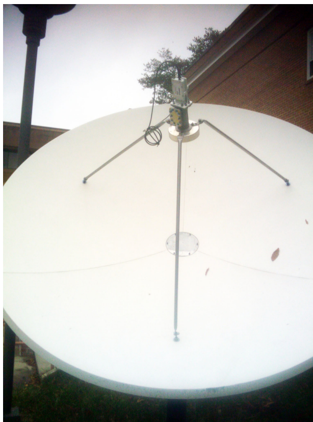
Photo of GNC-A dish installed at Bowie State University of Maryland, United States. The LNB shown attached to feed horn and properly mounted to reflector.
