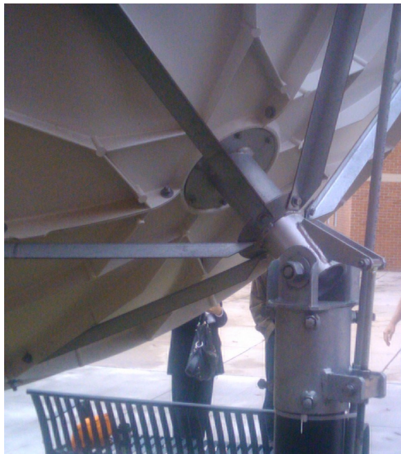
Back of the dish showing the support assembly attached to the canister and elevation assembly.
