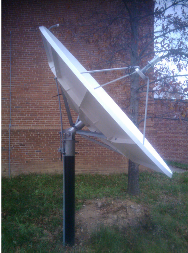
Installed GEONETCast Americas station at Bowie State University in Bowie, Maryland, USA. Profile shows reflector dish and focal point.
